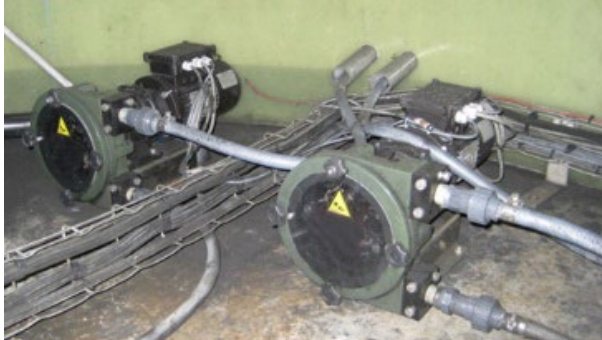
FRANCE: Transfer of lime milk or ferric chloride with Halar coated DFB 16
