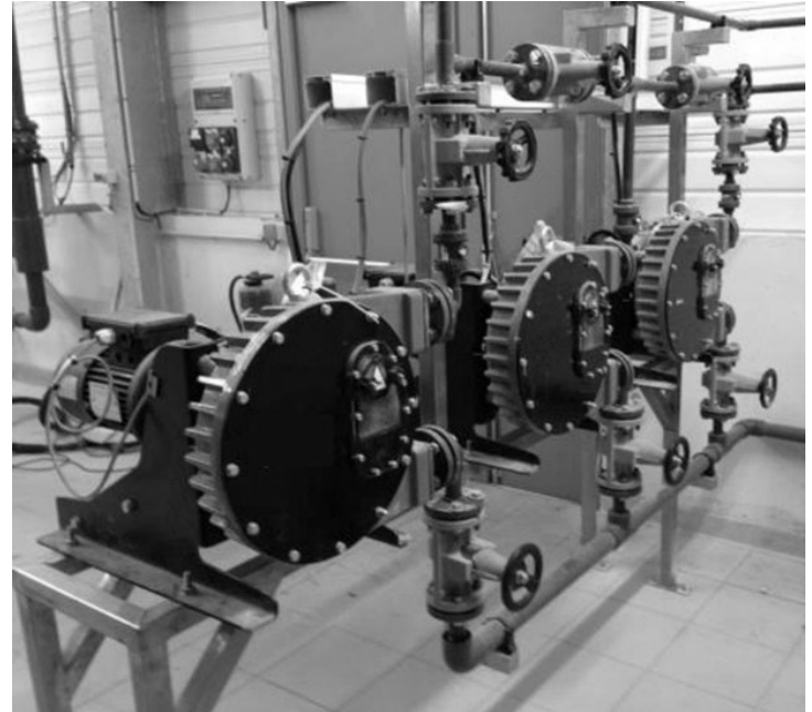
FRANCE: Dosing of activated carbon with DFD 25
